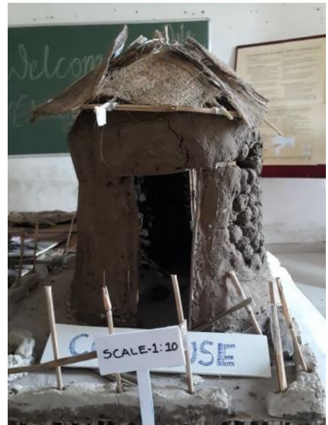
House model made with Cob Method
