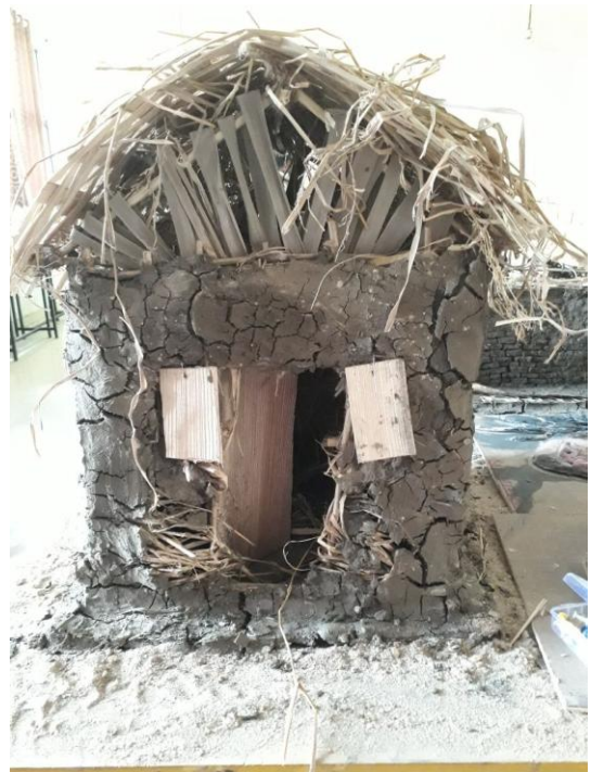
House model made with Wattle and Daub Method
